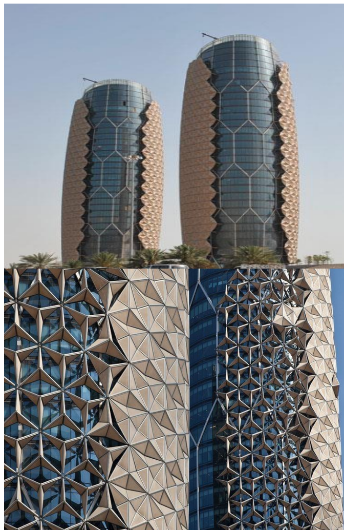
Al Bahar Towers designed by Aedas in Abu Dhabi, the double skins of the building is motivated by referring to the Institut du Monde Arab in Paris based on the objective of cooling and shading a building. (Source : The author).
