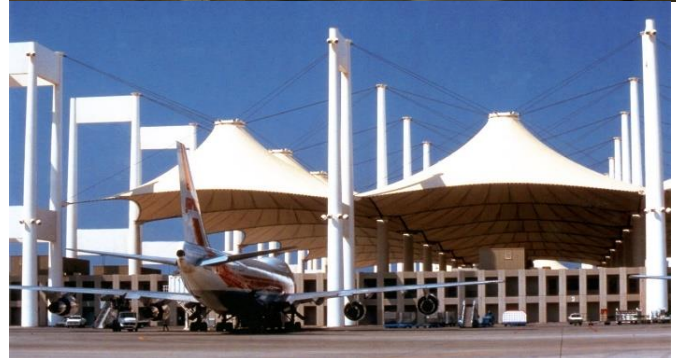
King Abdulaziz Hadj Terminal in Jeddah, designed by Owings & Skidmore; the material use for the membrane is Teflon coated fiber glass. It was the largest membrane using such material. The structure is referring to the tent and using a megastructure and for each membrane, they used four pylons and cables suspending the membrane. . (Source of the photos : Aga Kham Award website).
